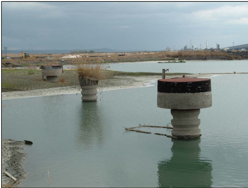
South Spillway Inlets - Before
