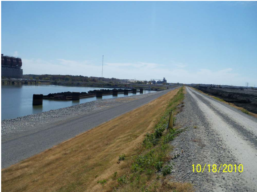
North East Dike - After
