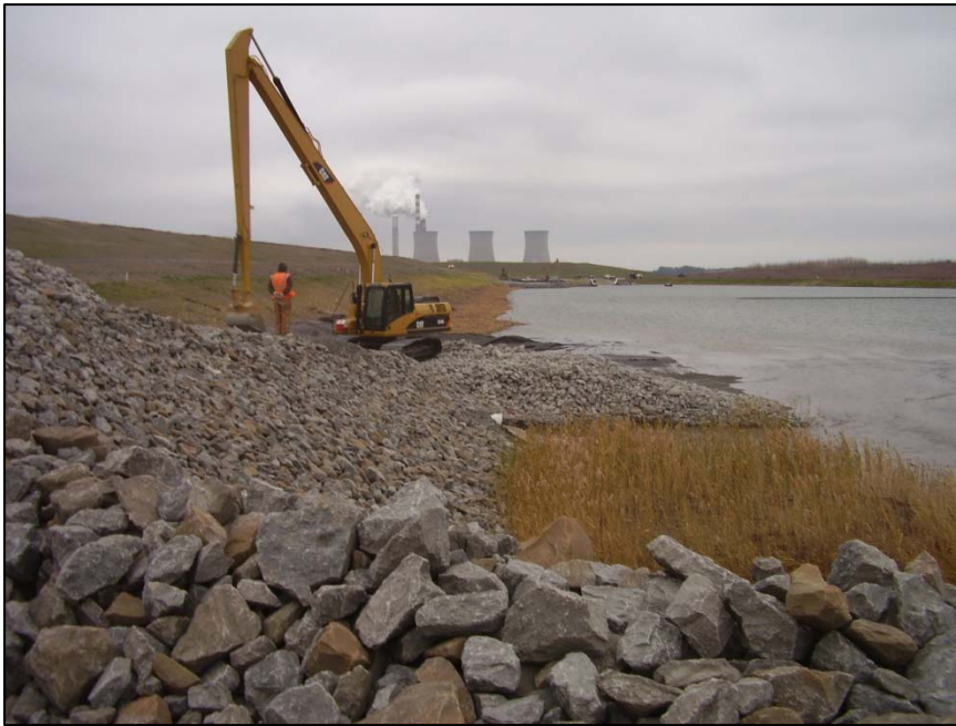
East Pond South Slope Buttress - Before
