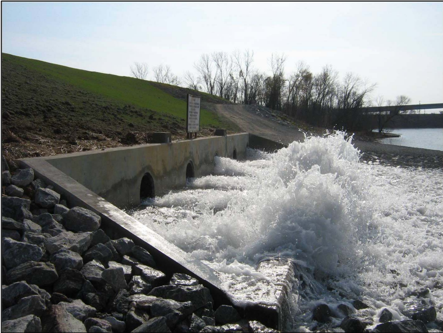
South Spillway Outlets - After
