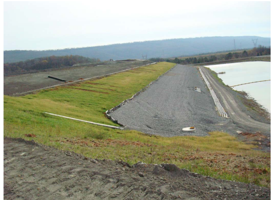
Gypsum Stack West Slope Buttress - After
