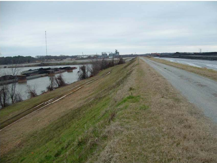
North East Dike - Before
