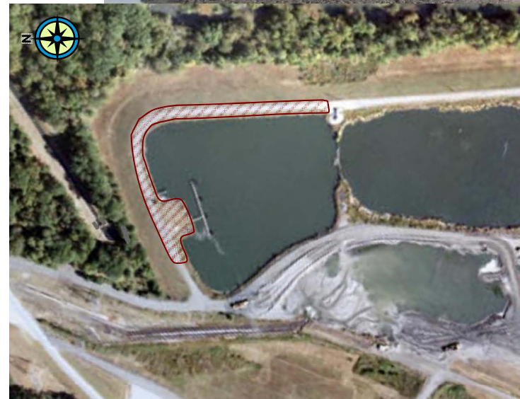
Colbert Bottom Ash Pond – Dike Lowering to Remove High Hazard
