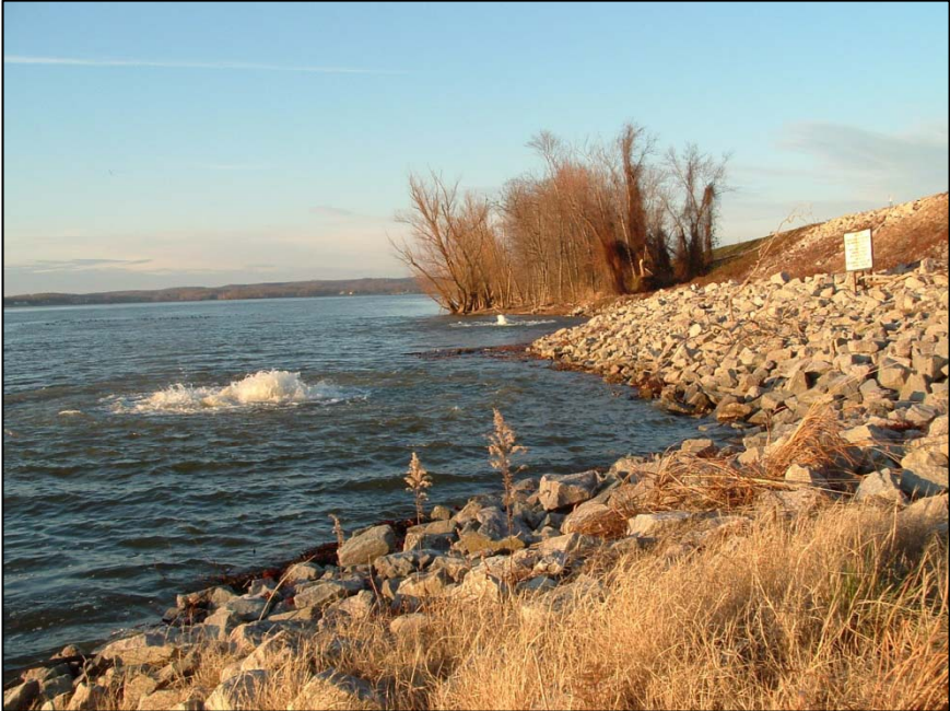
South Spillway Outlets - Before
