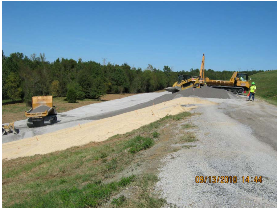
Gypsum Stack Seepage Drain and Armoring
