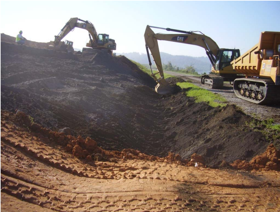
Slope and Drainage Improvements
