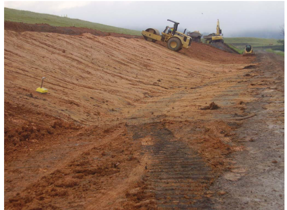
Slope and Drainage Improvements
