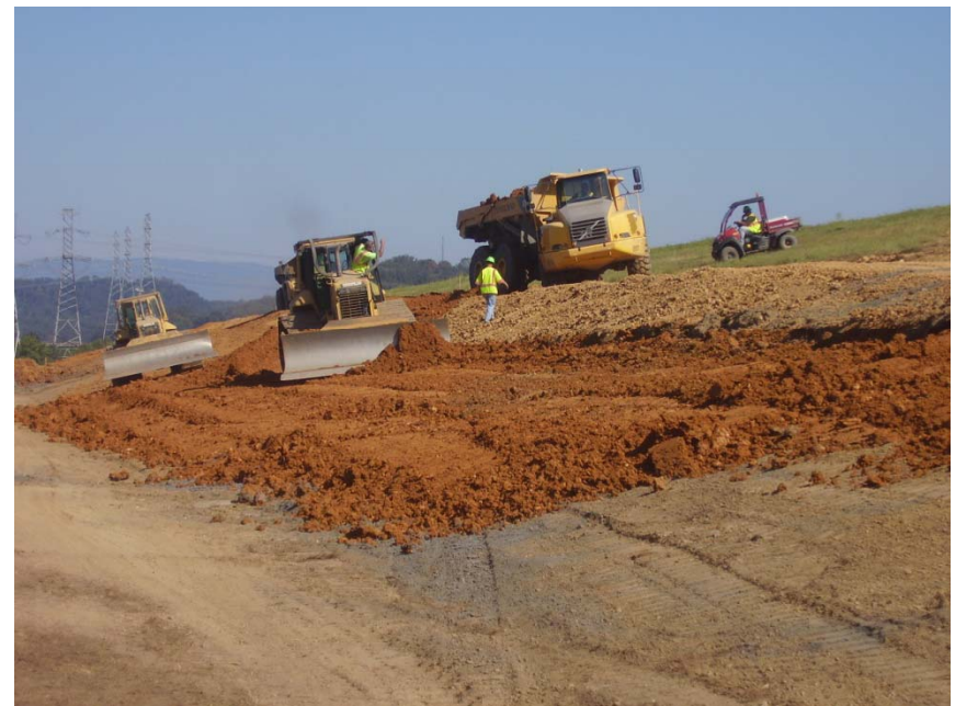
Construction of Improvements at Bull Run
