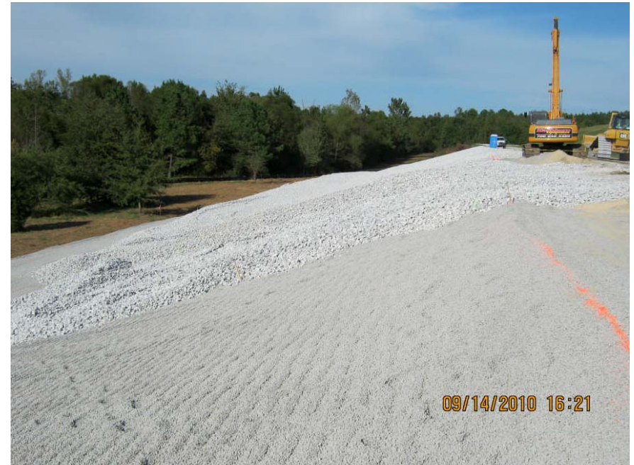
Gypsum Stack Seepage Drain and Armoring
