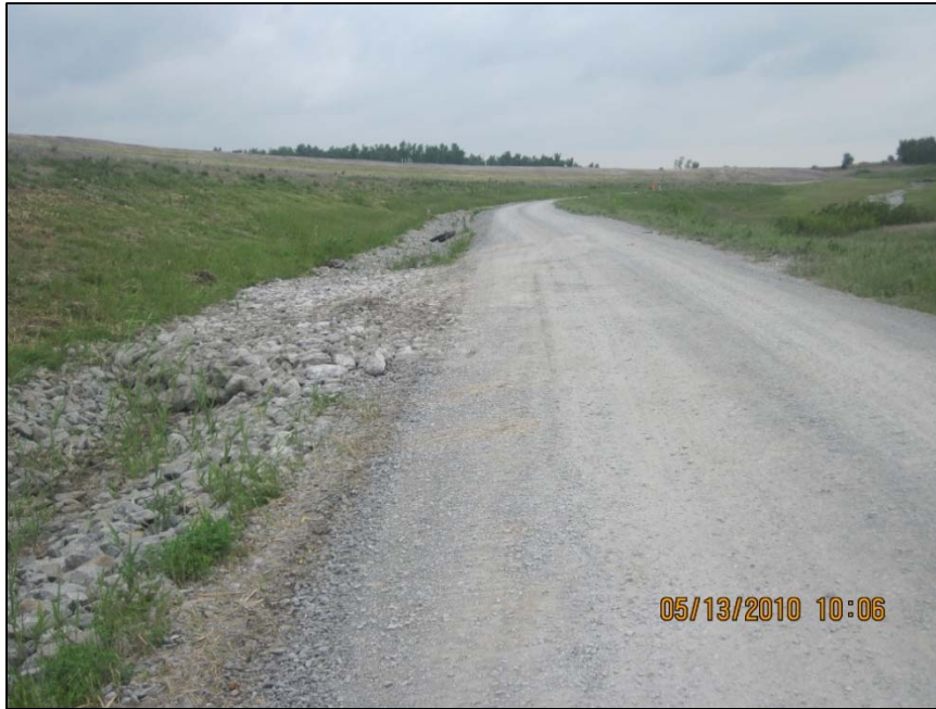
East Pond East Slope Armoring - Before
