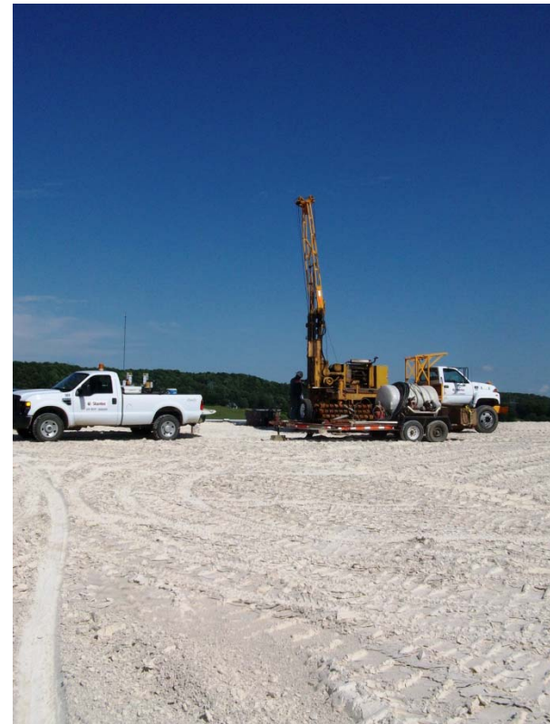
Geotechnical Drilling at Cumberland
