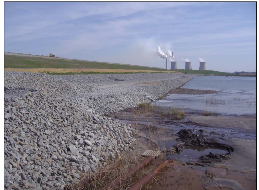
East Pond South Slope Buttress - After
