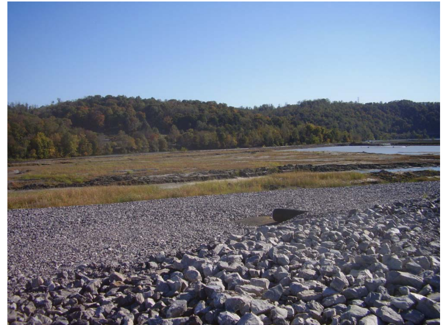
Gypsum Stack Buttress – After Pool Lowering
