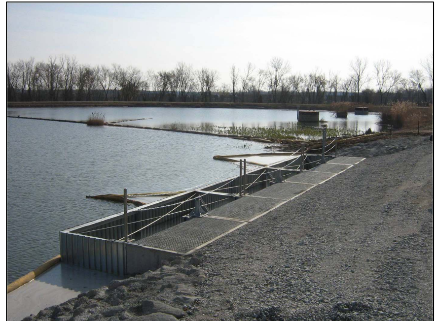
South Spillway Inlets - After
