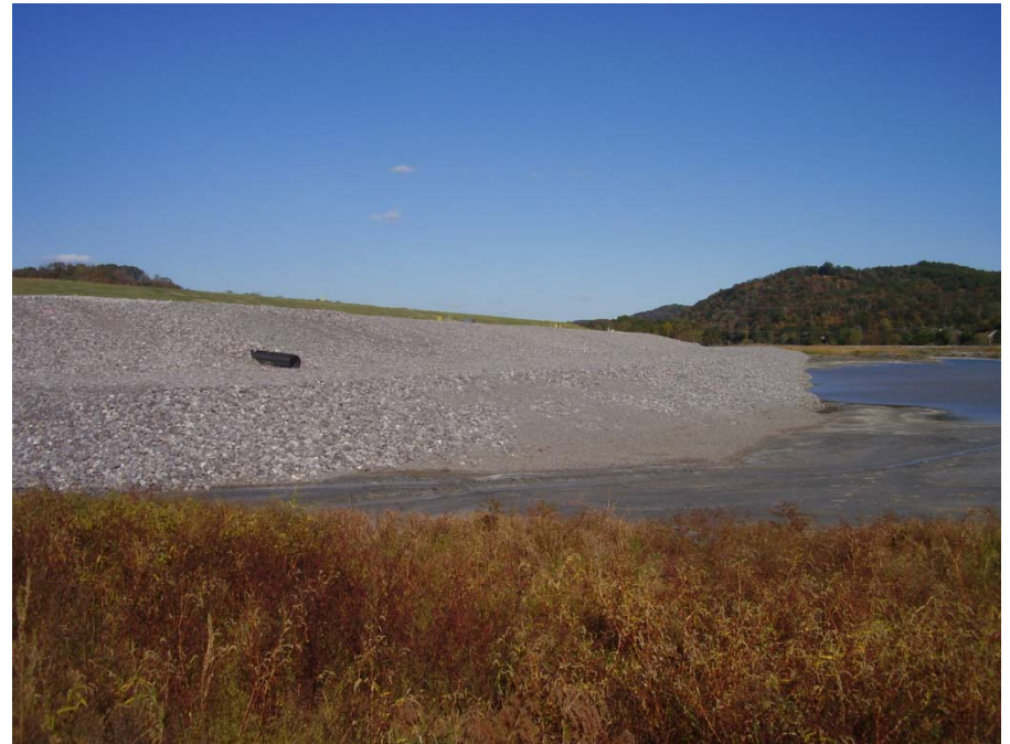
Gypsum Stack Buttress - After
