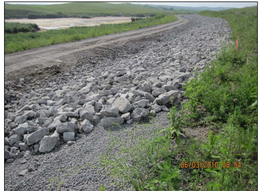
East Pond East Slope Armoring - After
