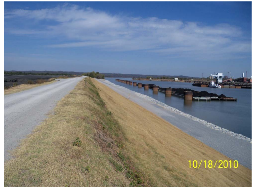
North East Dike - After
