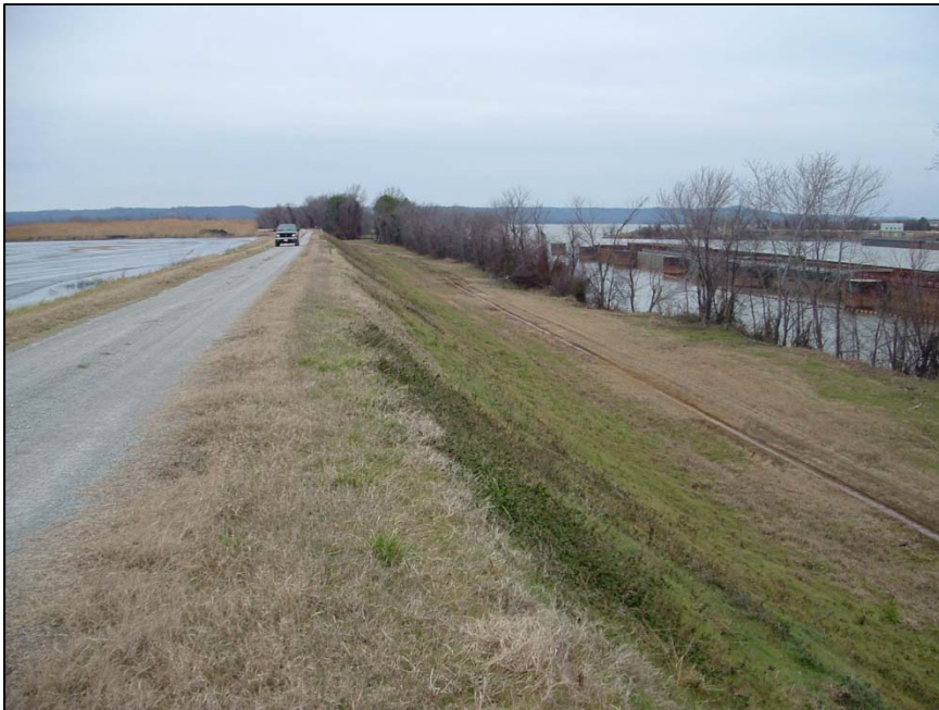
North East Dike - Before
