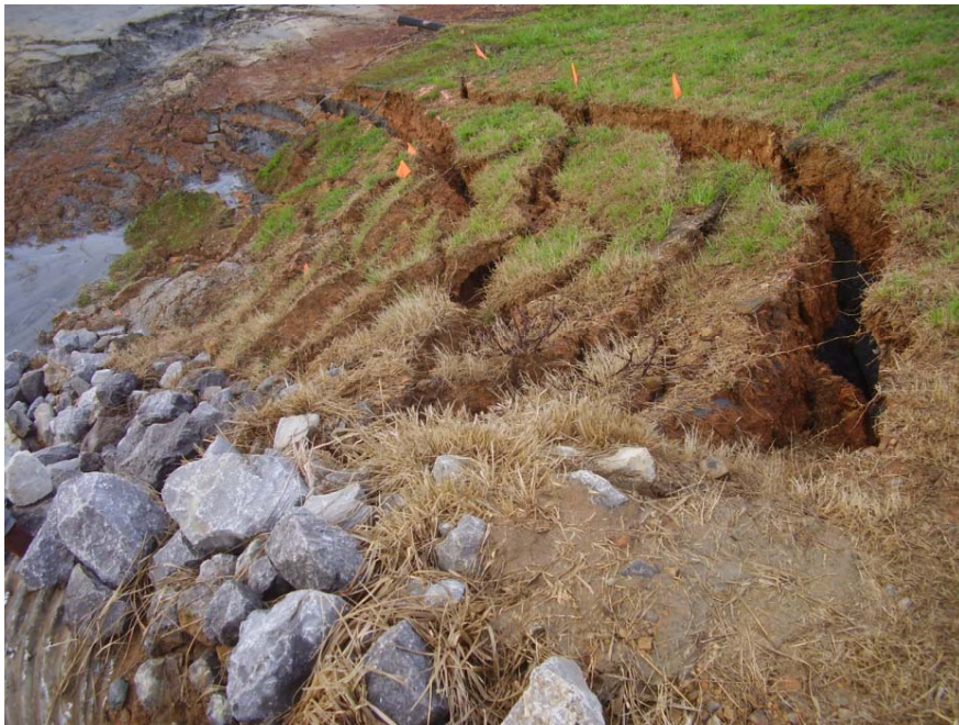
Gypsum Stack Buttress - Before
