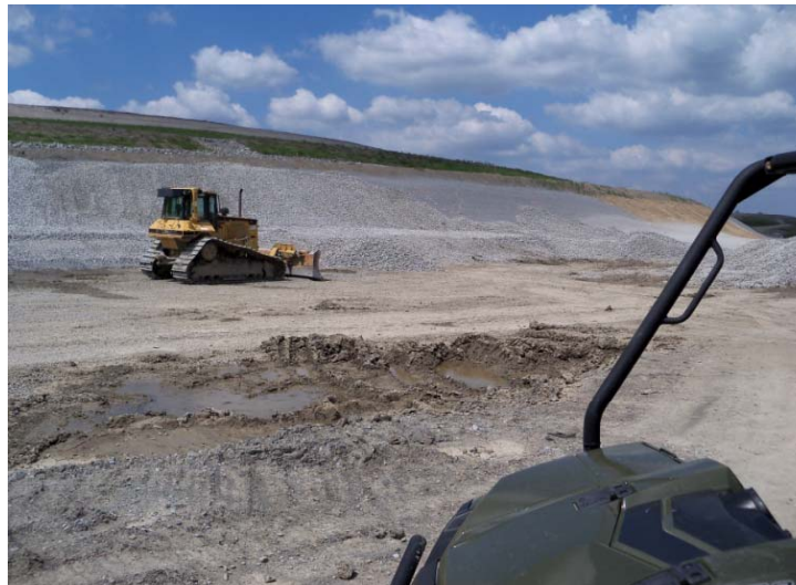
Paradise Scrubber Complex Armoring
