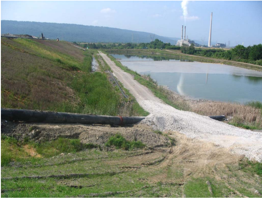
Gypsum Stack West Slope Buttress - Before
